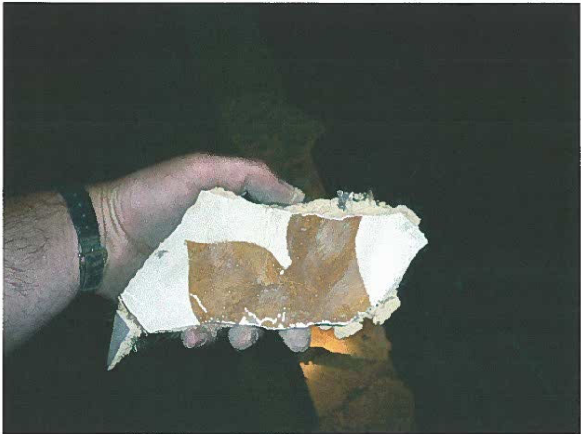
Picture 4 – Piece of original stencilled ceiling plaster
