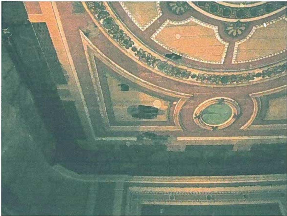
Picture 1 – Typical section of Theatre ceiling
