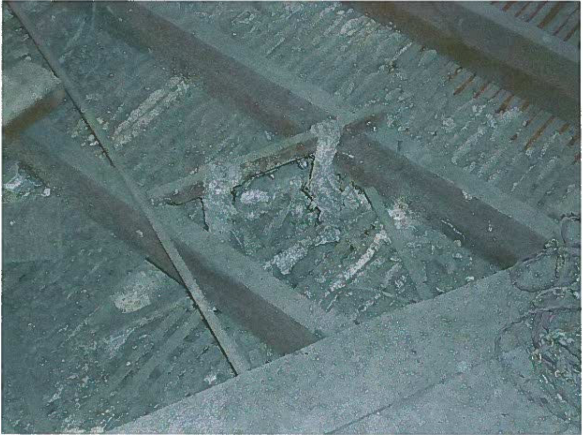
Picture 7 – Typical fibrous plaster support
