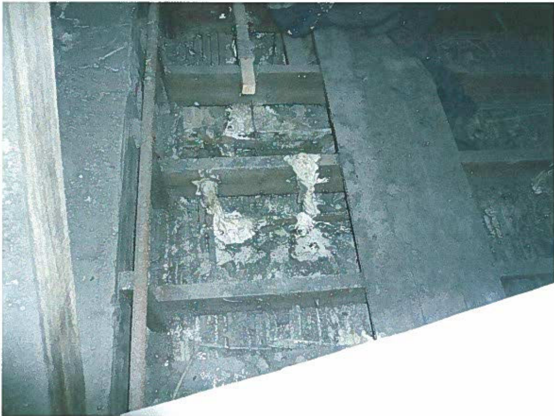
Picture 9 – Some later fibrous plaster supports
